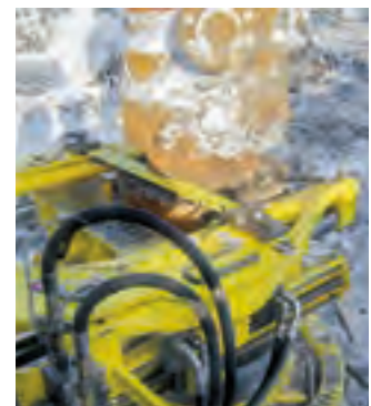
Guillotine cutting wellhead
