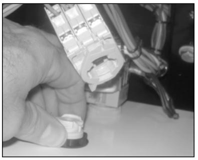
Figure 7-13. Remove the locking ring to take the front of the switch out of the control panel.
