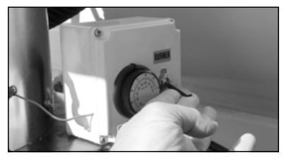
Figure 5-52. Push the power switch up to turn on the water heater.
