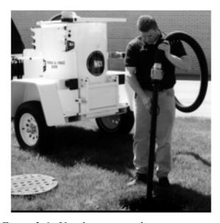
Figure 3-6. Use the suction tube to extract water and debris from the valve box.
