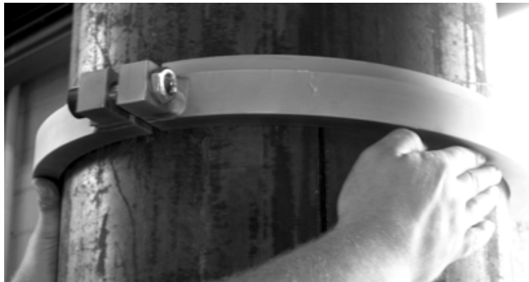
Figure 5-6. Hold both halves of the guide ring on the pipe and insert the screws through the brackets. Put the nuts on the screws.
