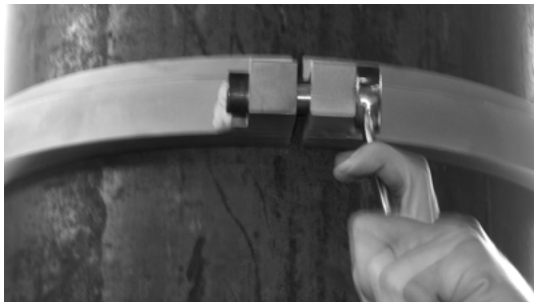
Figure 5-7. Tighten the nuts on the guide ring screws securely.
