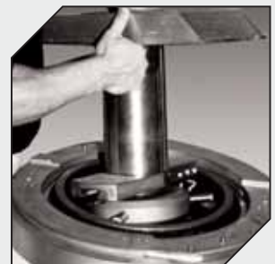
Perform internal casing cut and internal bevel.
