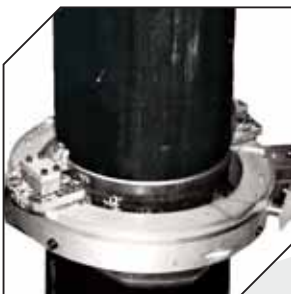
Sever the casing above the wellhead.
