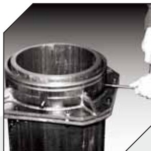
Remove Split Frame and install wellhead adapter ring.
