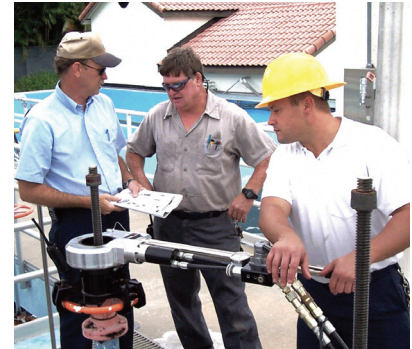
Figure 4 - RS-2 Hydraulic Exercising Water Treatment Valve
