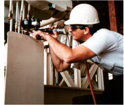
Figure 4 - Small split frames are used for socket weld removal
