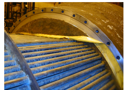
Figure 5 - Machining flange to restore tolerances and finish
