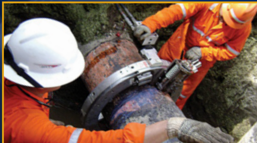
Split frames offer precision cuts important when making the "money cut"
