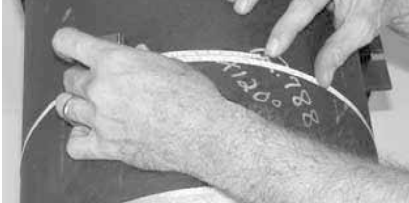
Figure 5-3. Verify the pipe circumference by measuring.
