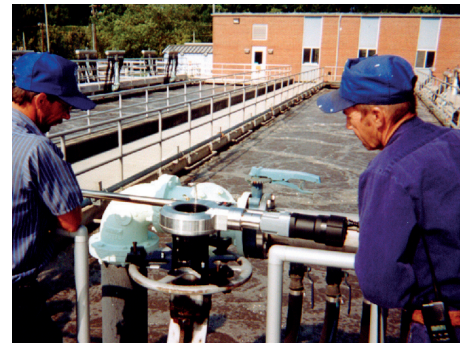
Semi or permanent mount universal handwheel adapters for any handwheel (two man operation shown)
