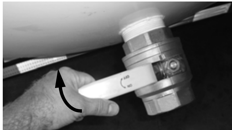
Figure 5-21. Close the tank drain valve.
