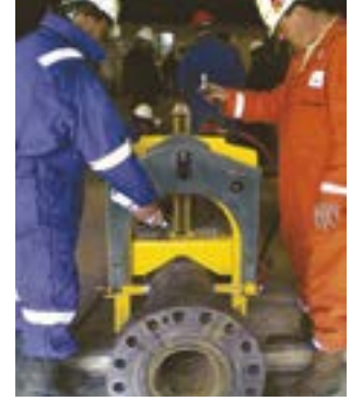
Guillotine cutting pipe
