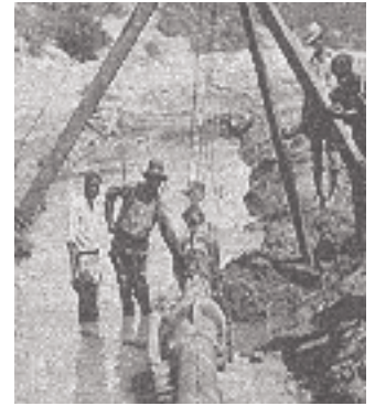
Early pipe fitting
