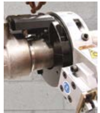
Socket Weld Removal
