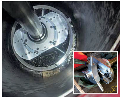
Figure 4 - Internal cutting module lowered to cutting depth
