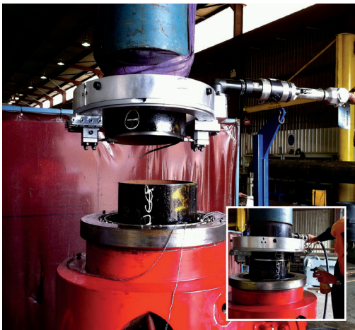
Figure 2 - EICC shown cutting the external conductor
