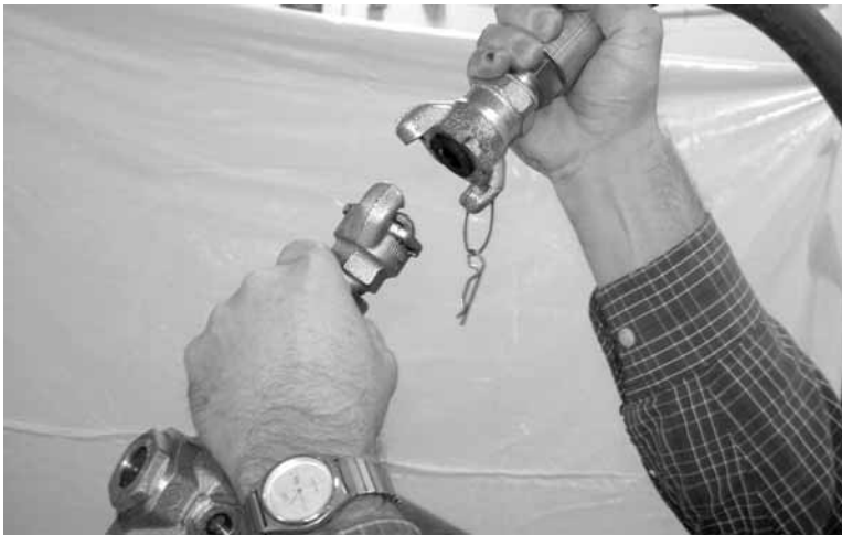
Figure 2-6. Disconnect pneumatic power by removing the air line from the pneumatic drive.
