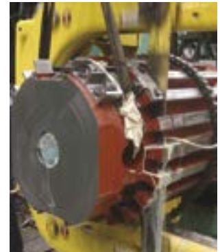
Guillotine Goliath cutting powerplant turbine shaft
