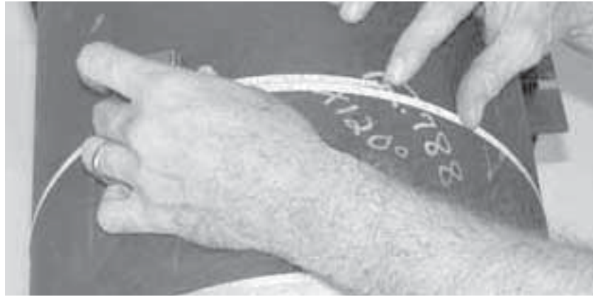
Figure 5-3. Verify the pipe circumference by measuring.
