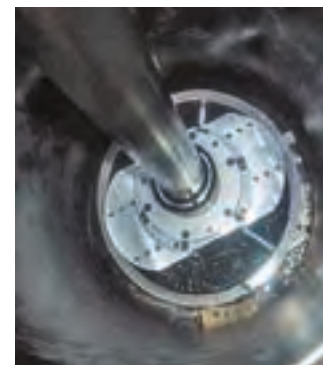
Internal cutting module lowered to cutting depth
